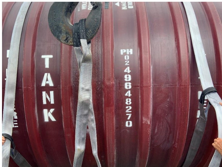
Picture 3 – Secure loose ends of the slings over the crane hook
