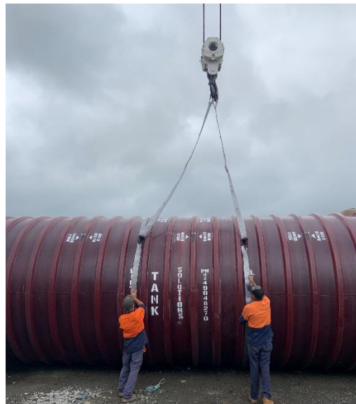
Picture – Adjusting the Choke Point
