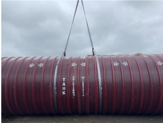
Picture 4 – Ensure an equal load on both slings
